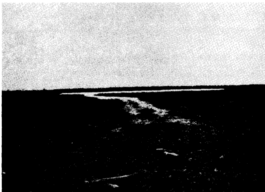
The Clam Shell Test Embankment FIGURE 24
