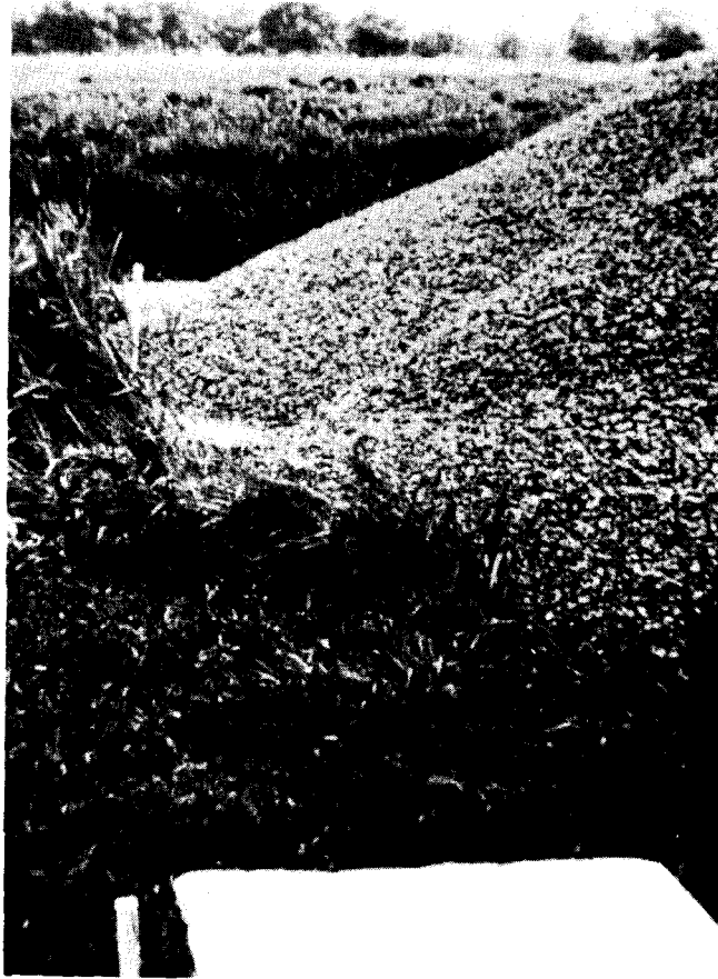
Settlement Plates FIGURE 10
